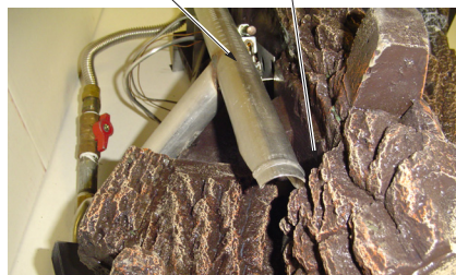
Figure 28A - Installing Middle Split Log Rear Top Side View
