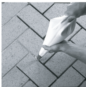
Figure 22 - Grouting Brick
