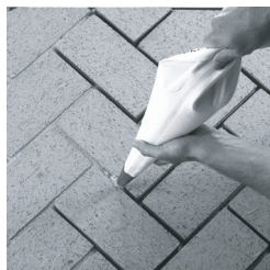
Figure 23 - Grouting Brick
